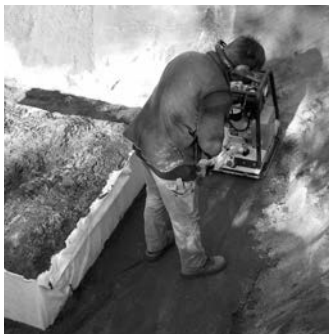
Compacting the work area
