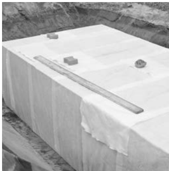
RAUSIKKO Box gravel trench with RAUMAT geotextile filter
