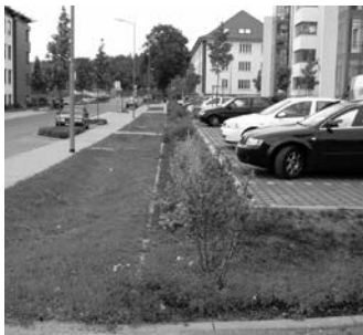
Percolation ditch of a ditch-gravel trench after completion
